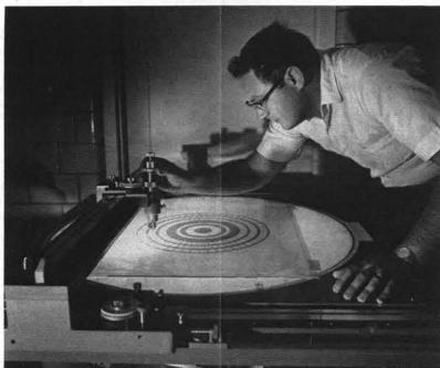
KARL D. SVENSSON (4411-5) uses this Swiss-made plotter to create a printed circuit master. The machine's extreme accuracy and rotating table are important tools in his cutting and stripping work on masters.
